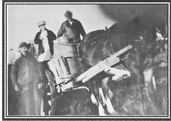
Clay was dug by hand and put into barrels. The barrels were pulled by horse in a cart up the bridge and the clay dumped from each barrel into the machinery.
